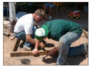
Repairing a sheep camp dwelling
