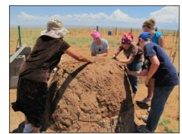
Fixing an adobe oven
